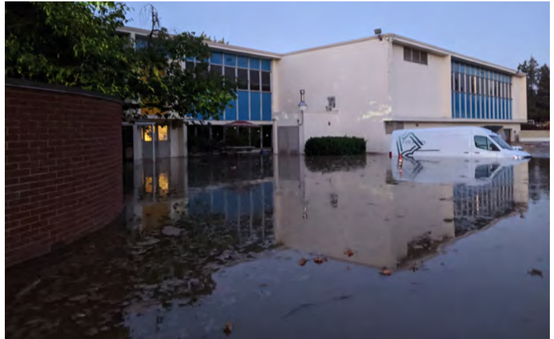
Reflected in our 2021 budget is repairs and recovery after a flood impacted our Operations Center last fall.
