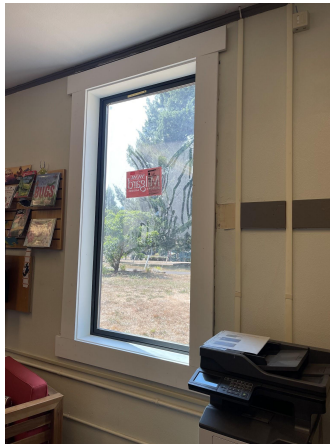
Parking lot and window upgrades
