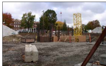
Photo of construction site taken Oct. 2009
