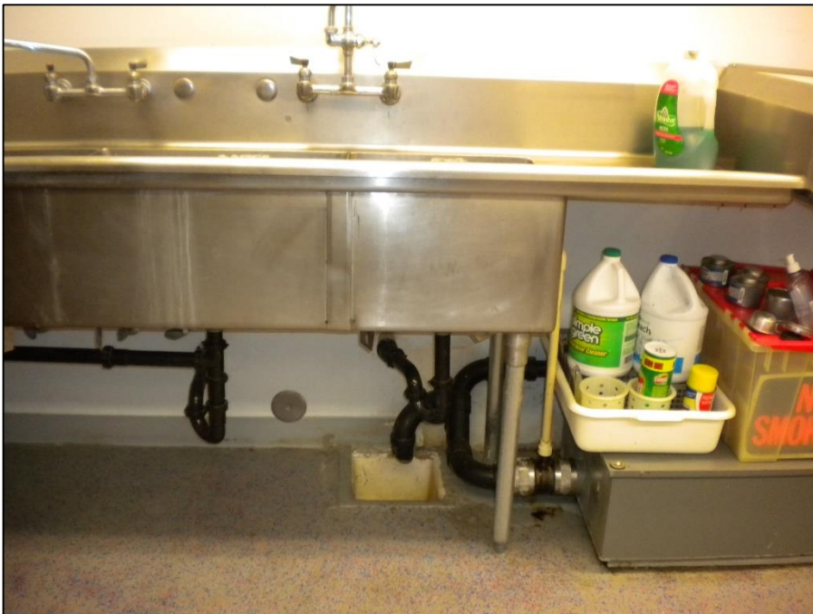
Photo 6: Kitchen sink and floor drain
