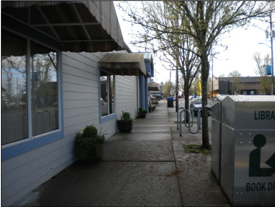
Photo 1: View of the front of the community center. Photo taken facing south
