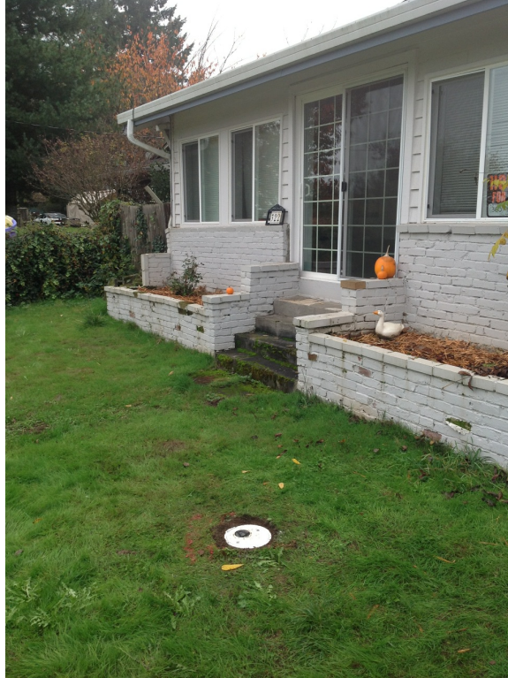
Photograph 13. Installed soil gas sampling port outside the residence at 322 N 1st Avenue, November 2012.
