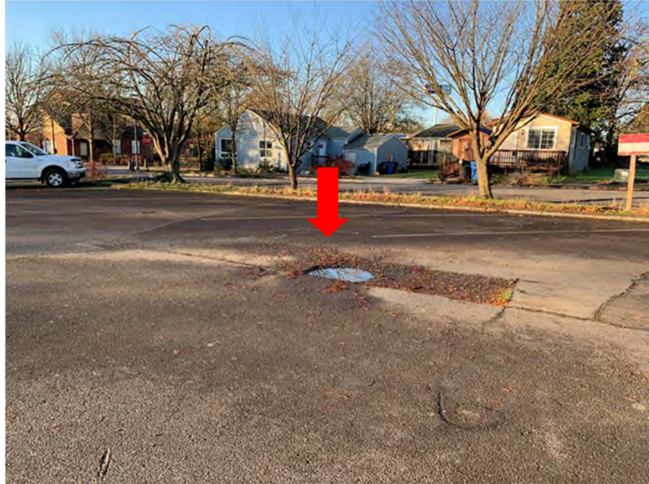
Photo 11. Portions of the concrete were cut and at the time of the site visit had standing water.
