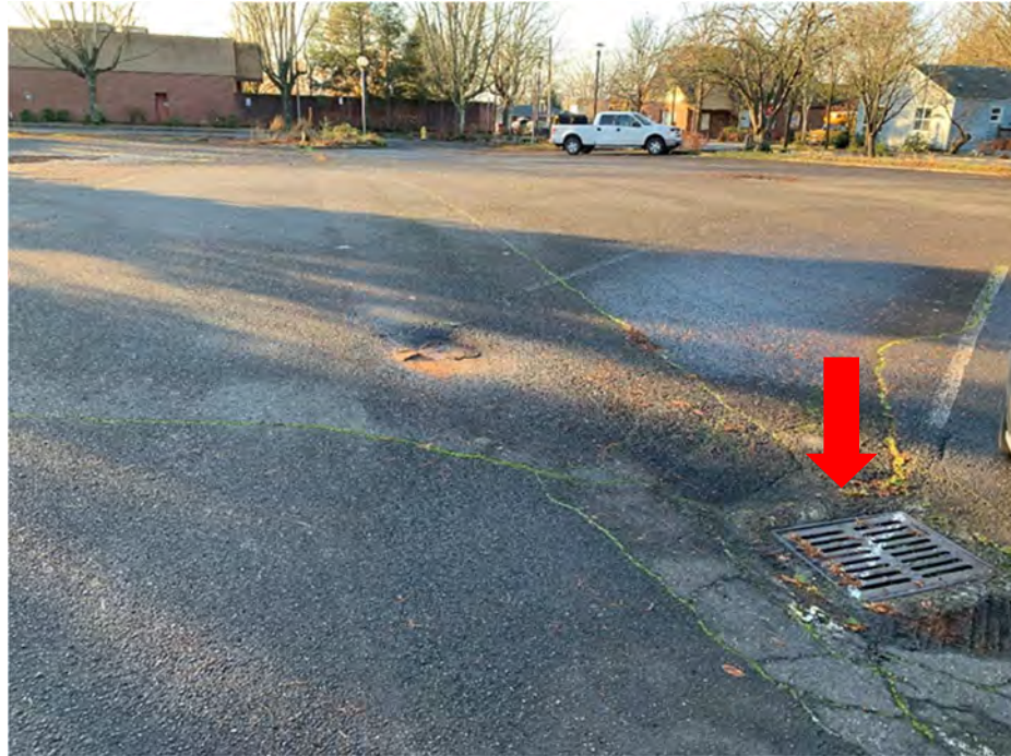
Photo 9. Looking south near the center of the property at a catch basin.
