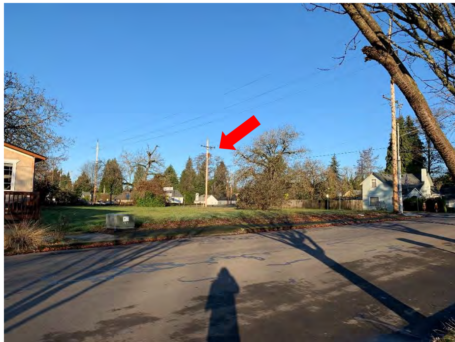
Photo 14. Looking west at a pole mounted transformer.
