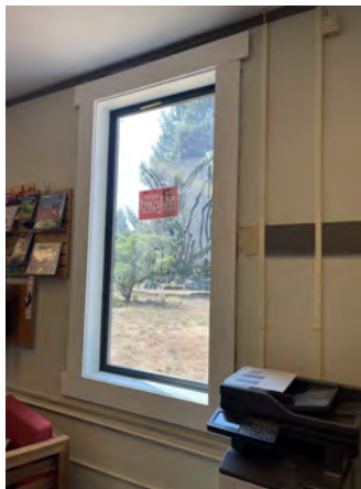
Parking lot and window upgrades
